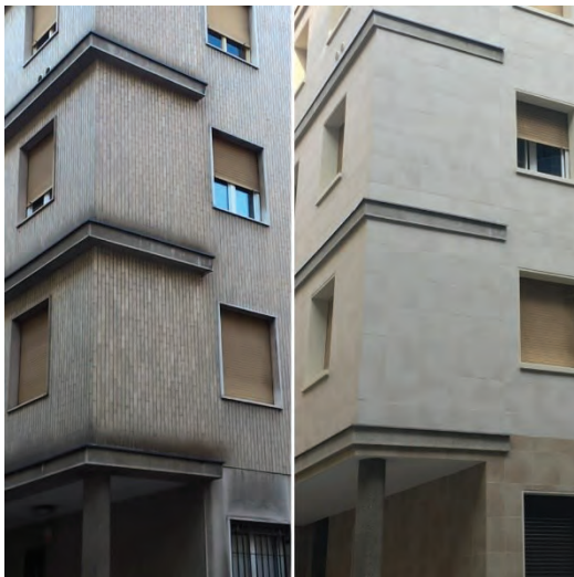
Figure 4: Private residential building pre and post retrofitting funded by Sharing Cities
